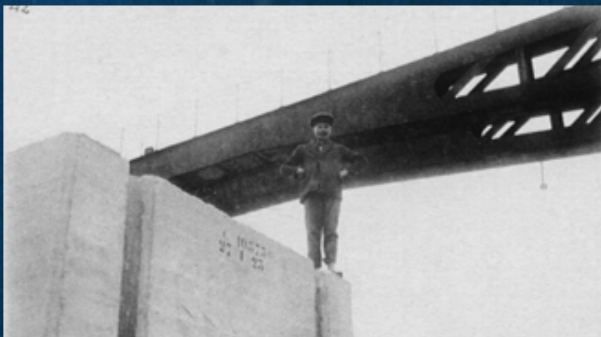
AYUB ON A CONCRETE BLOCK, WITH THE STEAM CRANE IN THE BACKGROUND.
